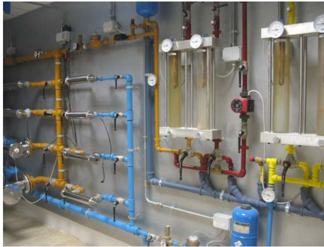
Figure 15 The installation for trials in the company
